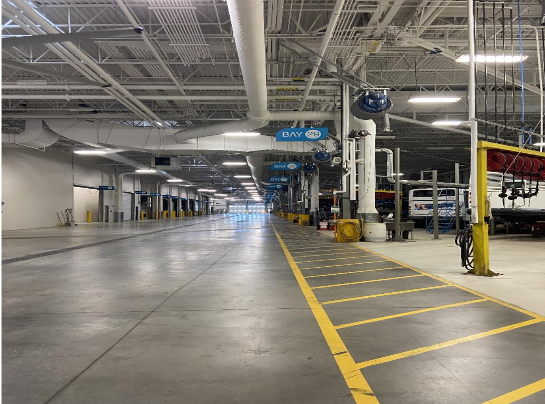
Garage where repairs and maintenance are performed – View 2
