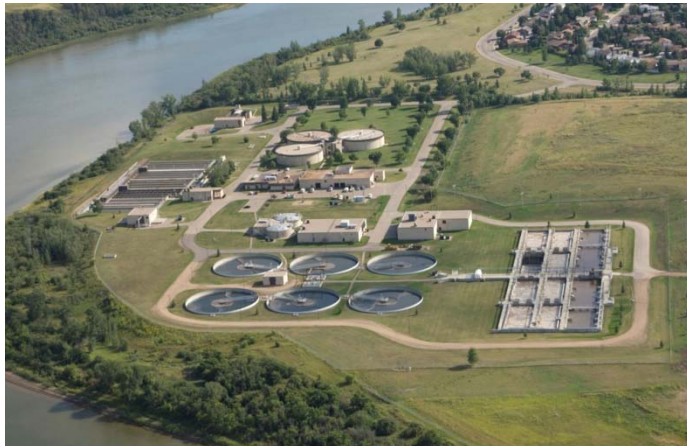
Aerial view of Wastewater Treatment Plant – Whiteswan Drive
