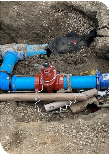
Valve and Pipe Installation
