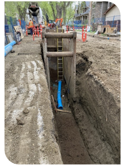
Water Main Installation
