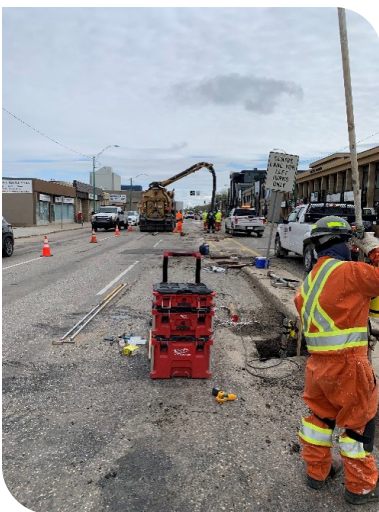
Anode Retrofit Installation
