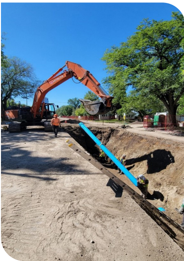
Water Main Installation
