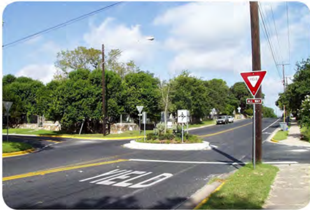
Traffic calming measures: Roundabouts.
