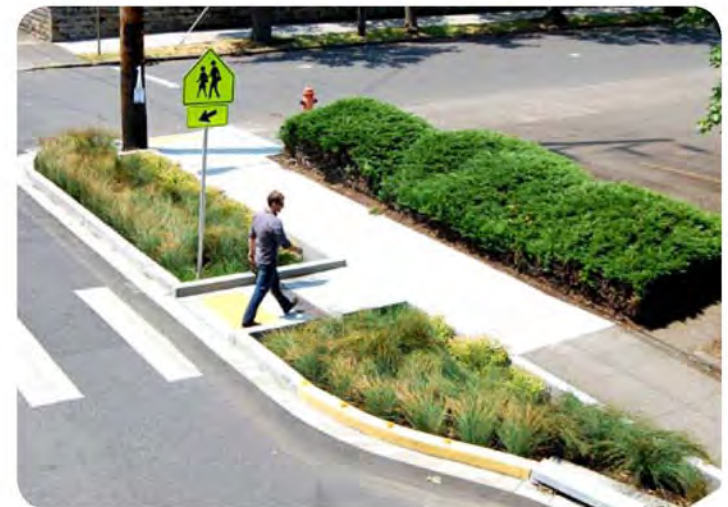
Bioswale stormwater management alongside a safe pedestrian crossing.
