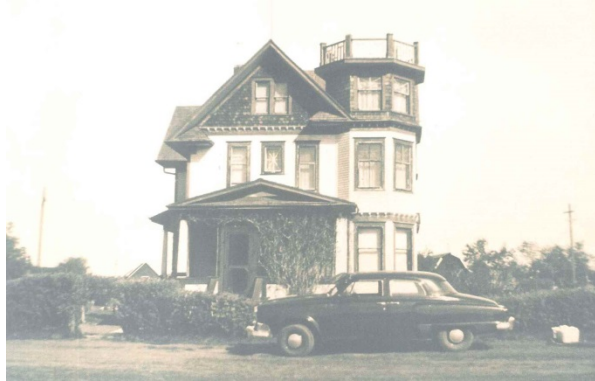
West Façade (1950s)
