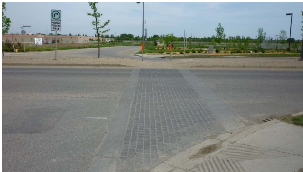
Exhibit 5-10: Textured Crosswalk using pavers at Stonebridge Boulevard and Wellman Crescent (Stonebridge)
