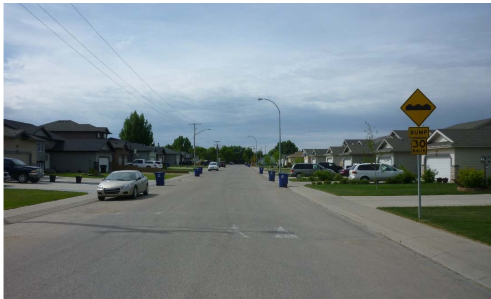
Exhibit 5-11: Speed Hump on Hughes Avenue (Dundonald)
