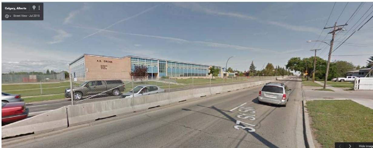
Exhibit 3: Raised Concrete Barrier and Fence on 37 th Street in Calgary
