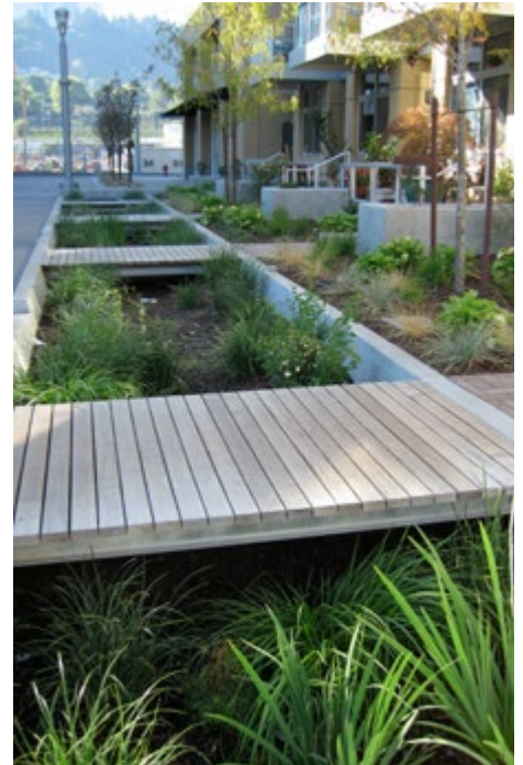
Figure 5.52 - Storm water swale at Dockside Green in Victoria
