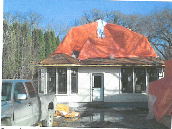
Rear (west))Exterior – March 2015
