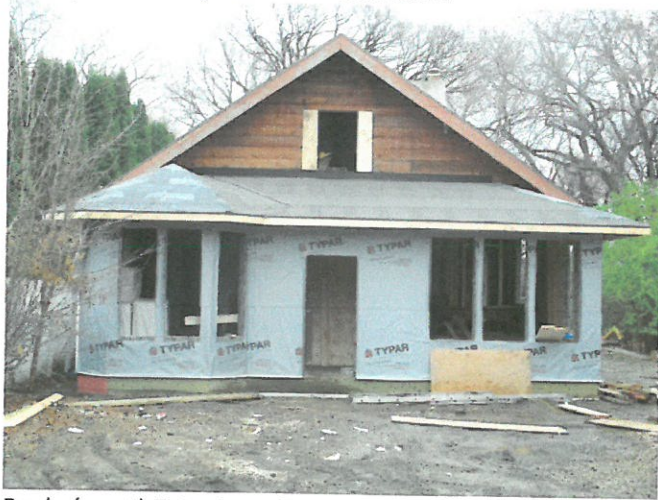
Back (west) Exterior - Nov. 2014
