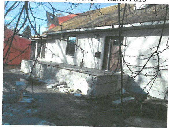
Side Entrance – March 2015
