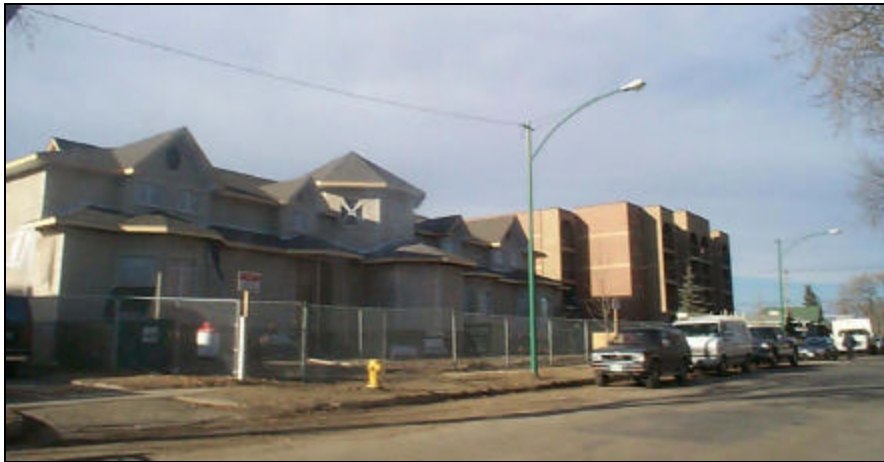
Convent under construction at 215 Avenue M South
