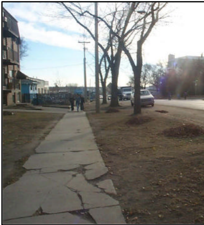
Sidewalk and boulevard on Avenue P
