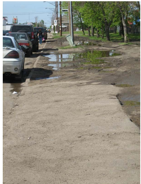
Central Avenue – East Side
