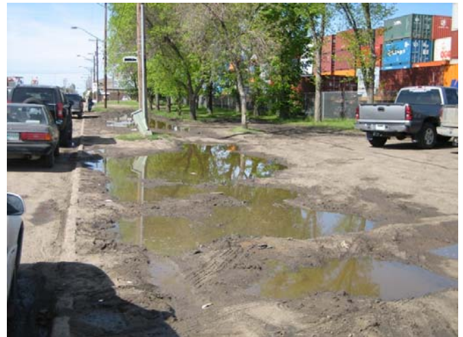
Inconsistent sidewalk treatment
