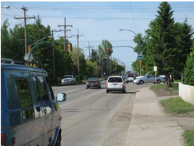
Central Avenue – Looking North
