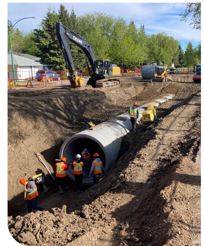
Installing Storm Sewer in W.W. Ashley District Park
