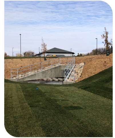
Churchill Park Dry Storm Pond Inlet/Outlet
