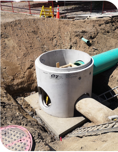
Manhole Under Construction near Churchill Neighbourhood Park
