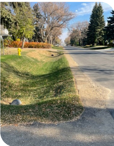
Montgomery Place Ditch and Culvert
