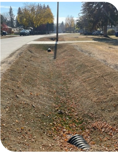
Montgomery Place Ditch and Culvert
