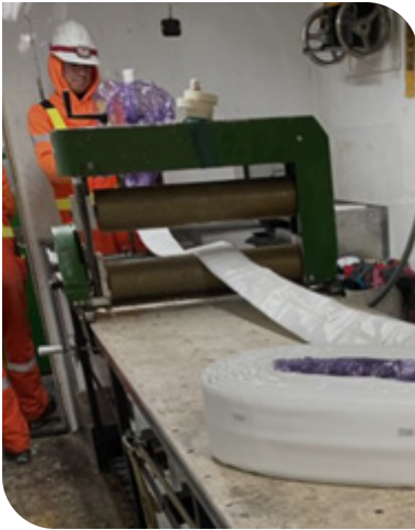
Sewer Lateral Liner Preparation
