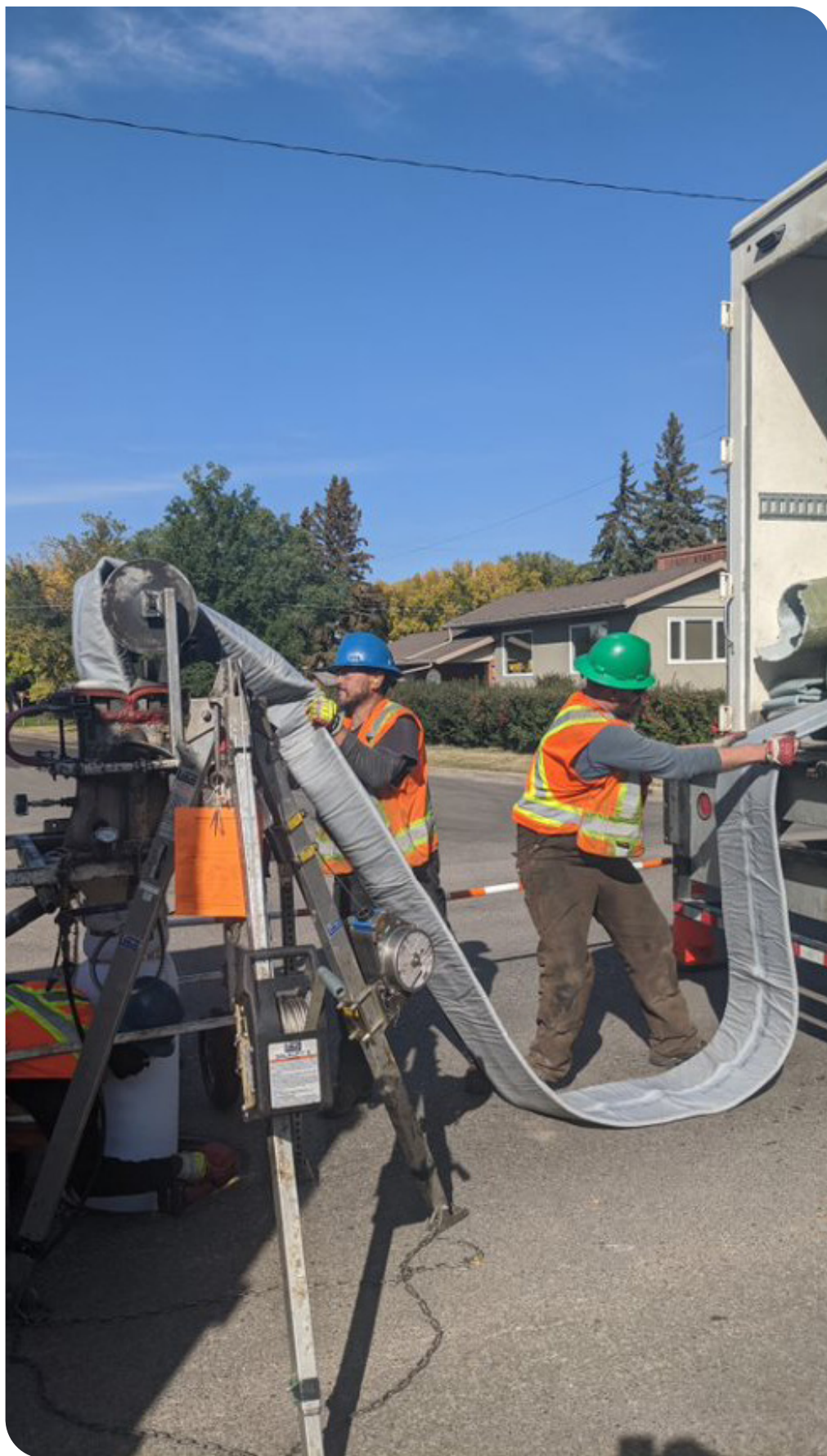
Sewer Pipe Maintenance
