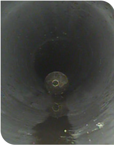
Sewer Main Liner Final Install
