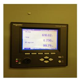
Monitoring equipment has been installed in 13 civic facilities to reduce utility costs and provide information that enables good management of facility equipment. The project involves installing a real-time data collection, reporting and analysis system that gathers utility consumption information from the facility. Industry research suggests that up to 5% utility cost savings can be achieved through utility monitoring.
