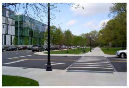
Figure 5.24 - Raised crossings along Forsythe Way in Boston
