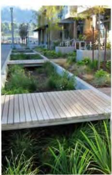
Figure 5.52 - Storm water swale at Dockside Green in Victoria
