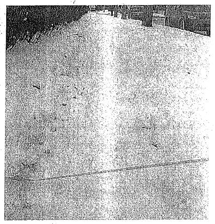
The adjacent picture is an example of a cleared compliant sidewalk. There is clear evidence that there has been an attempt to clear a path with a snow blower as is evident by uniform width which is approximately 1.2m. While there is some packed snow, the areas showing clear concrete is less than 3cm thick.
