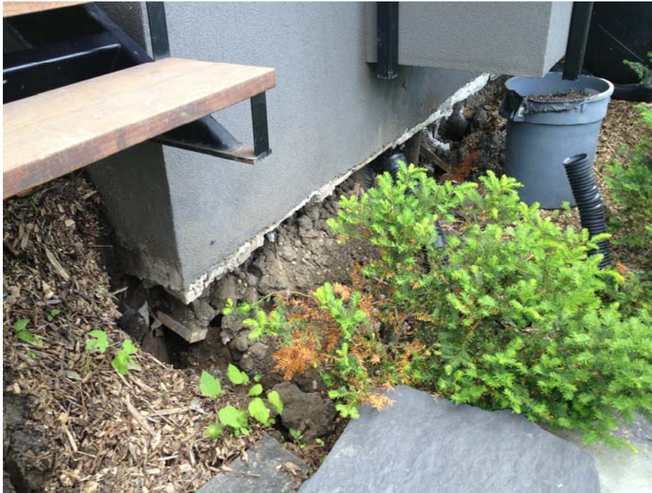
Photo C.13. Headscarp of East Failure in Backyard of 303 11th St. E.; Approx. 60 cm Drop (June 24, 2013)
