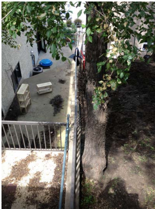
Photo C.26. Looking North at Concrete Retaining Wall between 230 & 306 Sask. Cres. E. (July 7, 2013)
