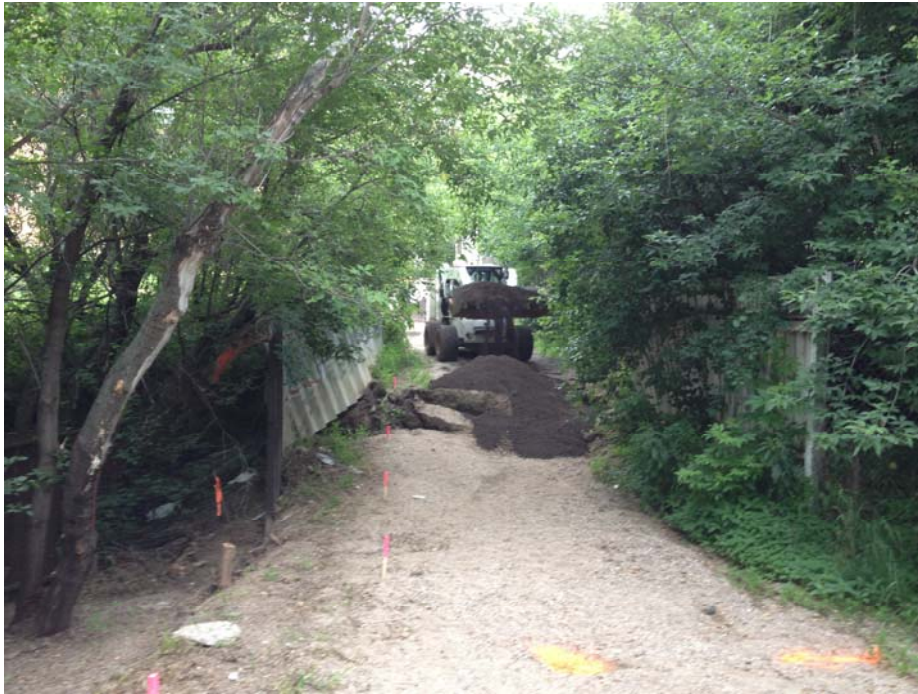
Photo C.21. Looking East at Public Works Filling Cracks and Regrading Lane (June 5, 2013)
