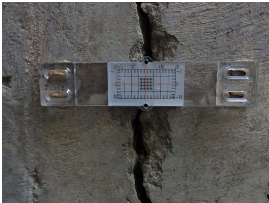
Photo F.2: Crack Meter Located on the Retaining Wall Behind 306 Sask. Cres. E. (CM1) (Sept 18, 2013)
