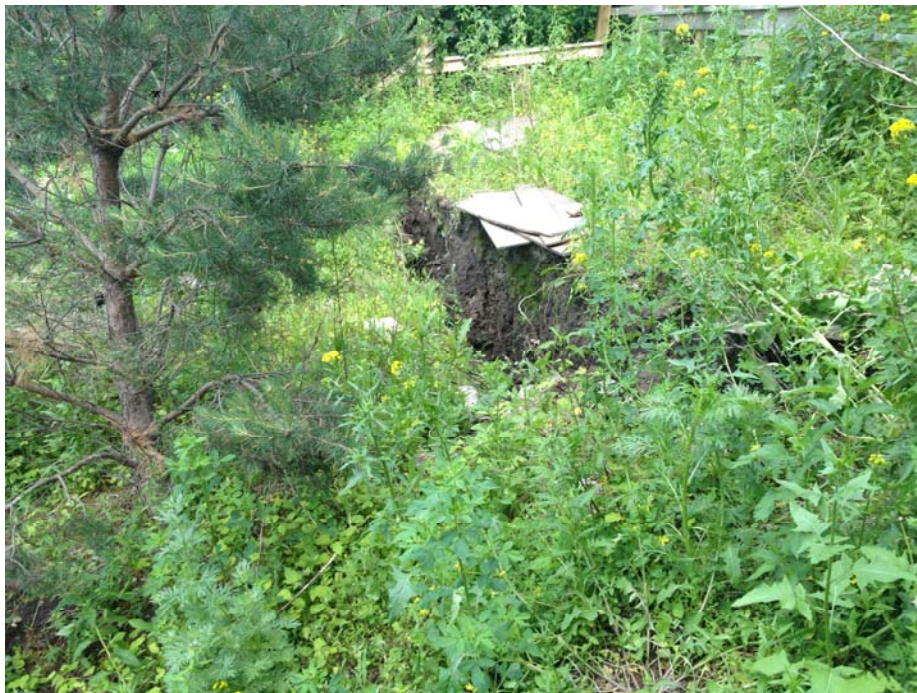
Photo C.12. Looking East at Headscarp of East Failure in Backyard of 305 11th St. E.; Approx. 90 cm Drop (June 24, 2013)
