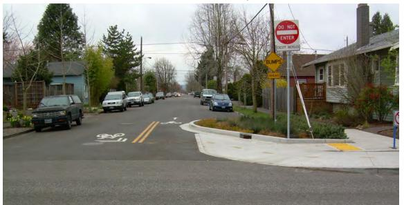
An example of a directional closure. The curb blocks one lane of traffic from proceeding through the intersection.
