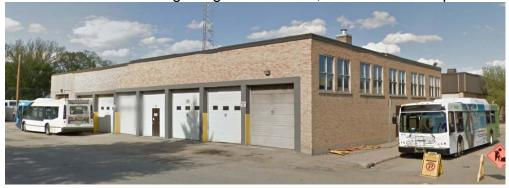
Parcel E – 1973 Building: Can be reused with strengthening of roof trusses.
