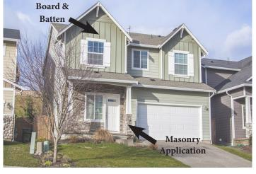
features near the garage edges, with the balance of the facade consisting of cement fiber siding.
