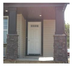
Wide-based columns, with stone detailing.
