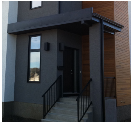
Covered entry feature, with supporting column.
