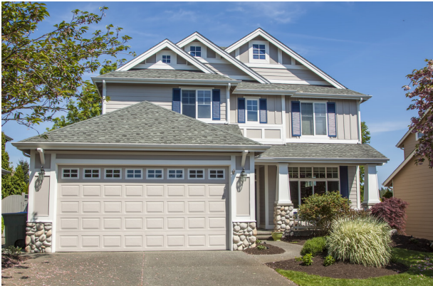
The attached garage projects 2.0 metres from the second storey of the dwelling.
