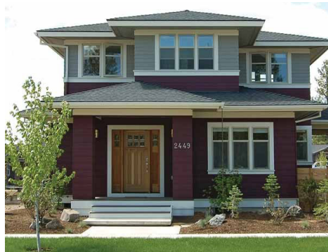
The use of a low-pitched hip roof, with wide overhanging eaves in a prairie style home.
