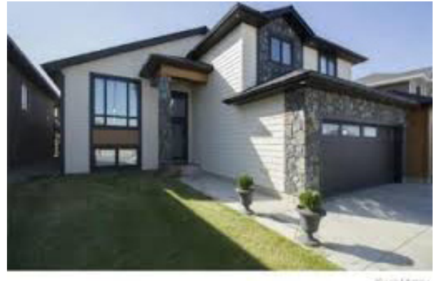
The attached garage projects 2.4 metres from the second storey of the dwelling.
