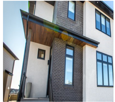
Covered entry feature, with supporting column.
