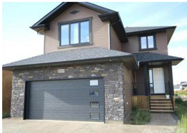
The attached garage projects 2.4 metres from the second storey bonus room.
