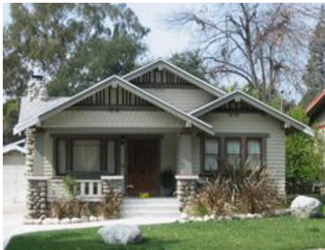
The use of a low-pitched gabled roof for a craftsman style home.
