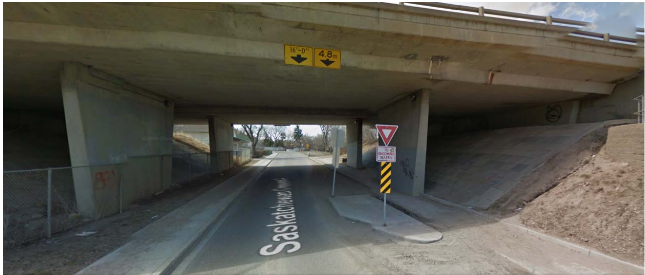
Exhibit 4-1: Existing Pinch Point beneath Senator Sid Buckwold Bridge (looking west)
