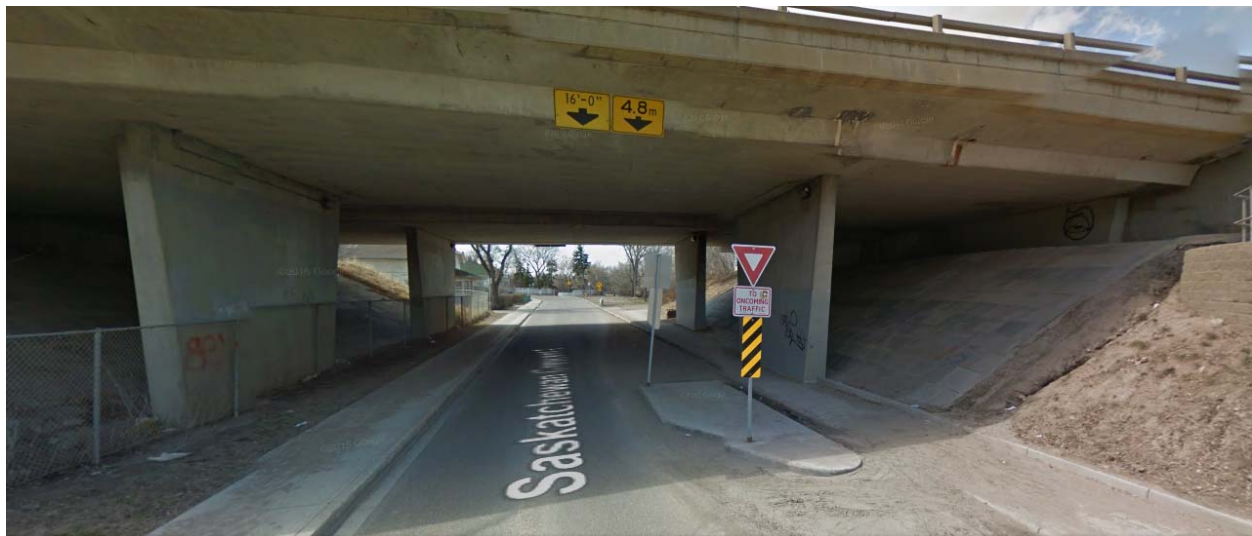
Exhibit 1: Looking West beneath the Senator Sid Buckwold Bridge
