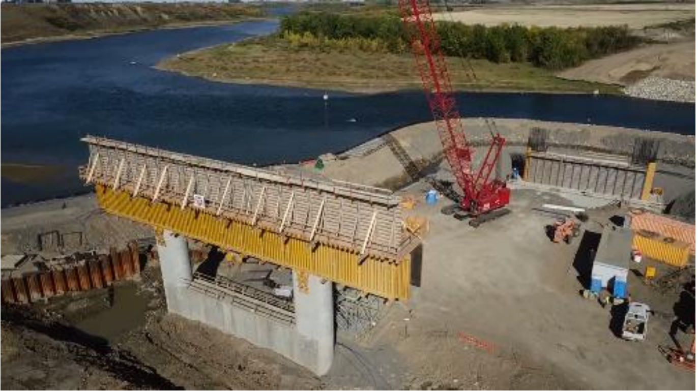
NCP Pier 1 & 2 (Early September 2016)
