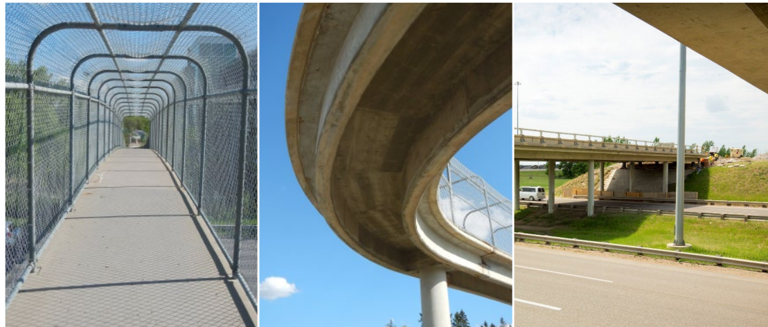
Pedestrian Overpass from 23rd Street to 21st Street over 22nd Street
