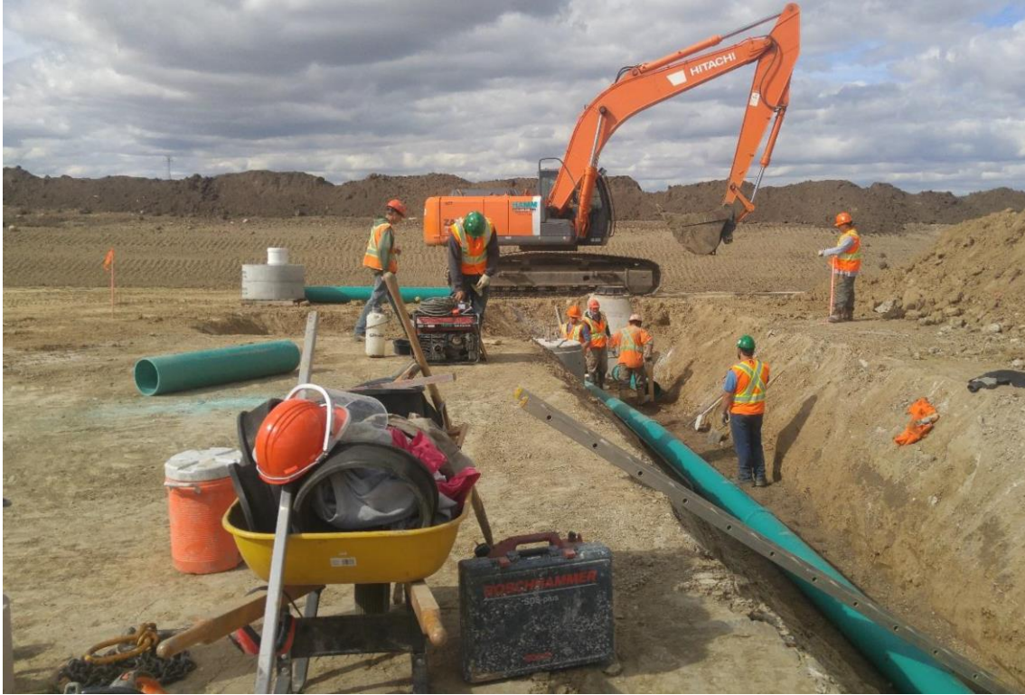
Storm Sewer Construction
