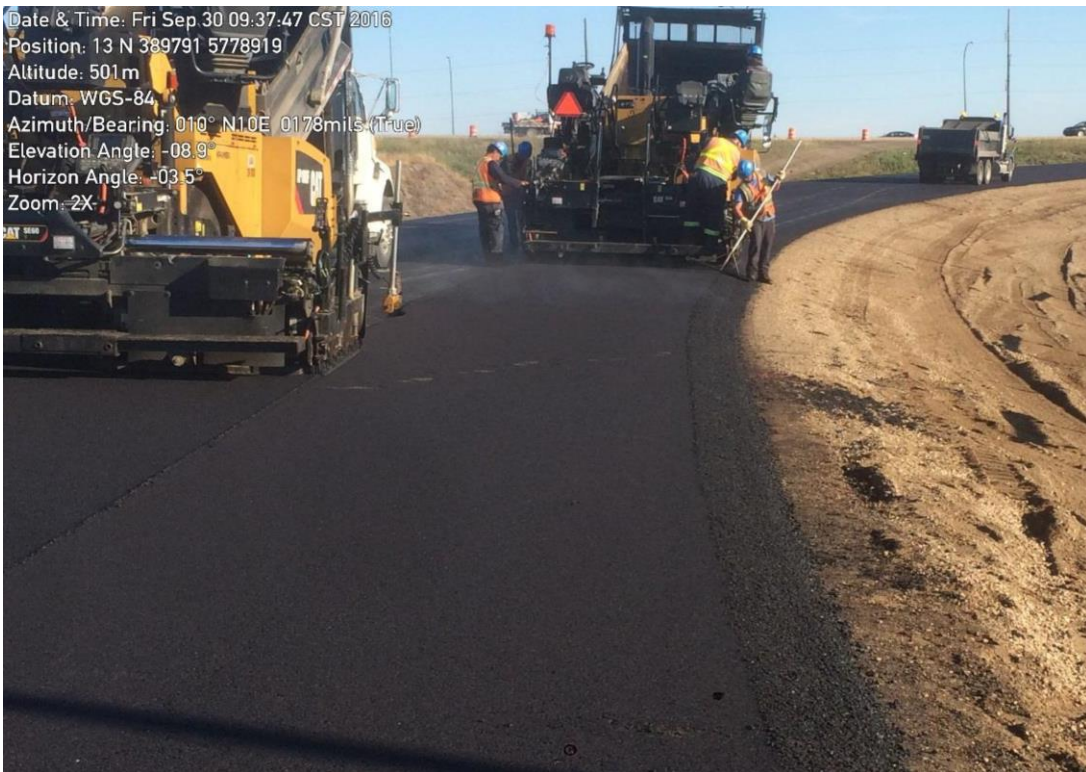
Circle Dr Offramp Bottom Lift Paving
