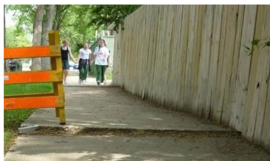
Repair - Grinding or Saw Cut
