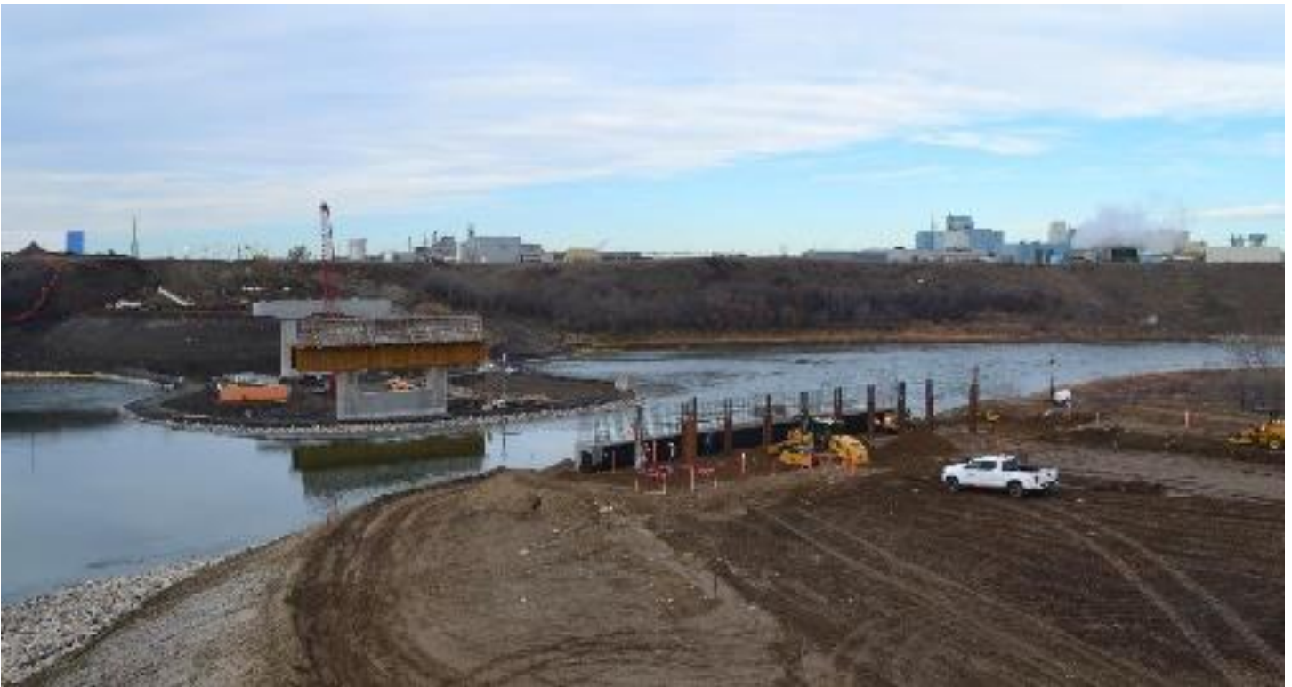
NCP Bridge – Pier 2 Cap Underway
