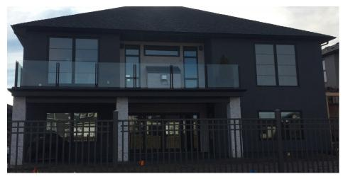
The area of the rear elevation (minus window area) totals 270 square feet. 90 square feet of stone has been provided, which satisfies the secondary material requirement. 140 square feet of window placement has also been provided, which satisfies the window and/or door placement requirement on highly visible lots.
