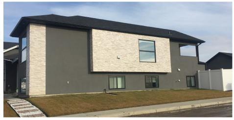
The area of side wall (minus window area) totals 300 square feet. 100 square feet of stone has been provided, which satisfies the secondary material requirement. 40 square feet of window placement has also been provided, which satisfies the window and/or door requirement on highly visible lots.
