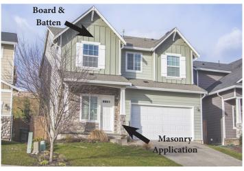
This home features board and batten siding along the dormers, stone accents along the veranda columns, with the balance of the front facade consisting of cement fiber siding.
