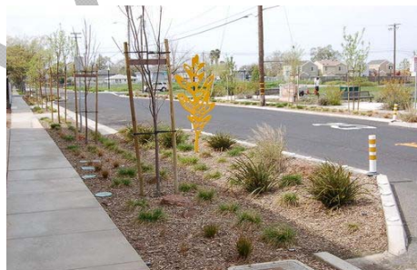
Figure 10: Stormwater bump out example
