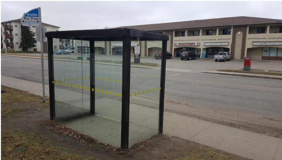
Bus shelter on Avenue W at 18 th Street
