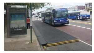
Transit platforms provide a raised landing area for passengers boarding and alighting transit. The platform eliminates grade changes for pedestrians, while proving a ramp on either end to accommodate cyclists passing over the platform. Shown is a temporary transit platform.
