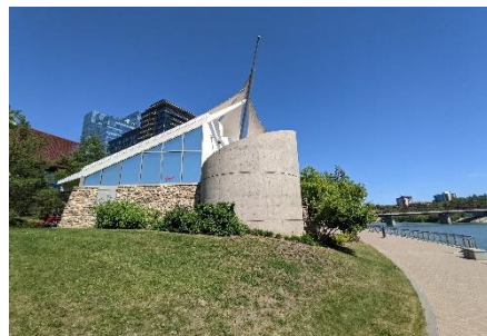
Looking east towards the River Landing Pavilion Building
