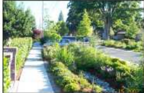
Surface runoff from the street is captured in a naturalized swale.
