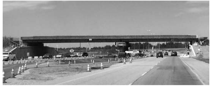
Boychuk Drive / Highway 16 Interchange Project Construction Tentative Completion July 31, 2019
