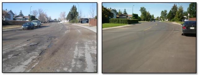
Figures 17 & 18: Collector Before and After 2012 Ultra Thin Overlay
