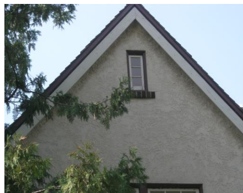
Steeply Pitched Roof (2014)
