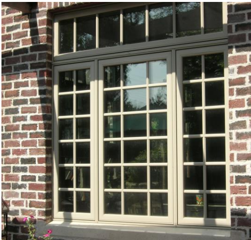
Brick Exterior with Tall Narrow Windows (2014)
