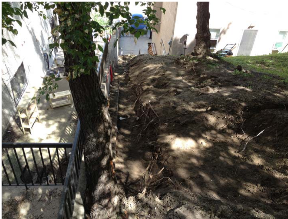
Photo C.28. Looking North at Partially Filled Trench (July 17, 2013)
