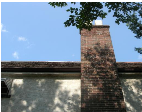
Chimney with Decorative Chimney Pots (2014)
