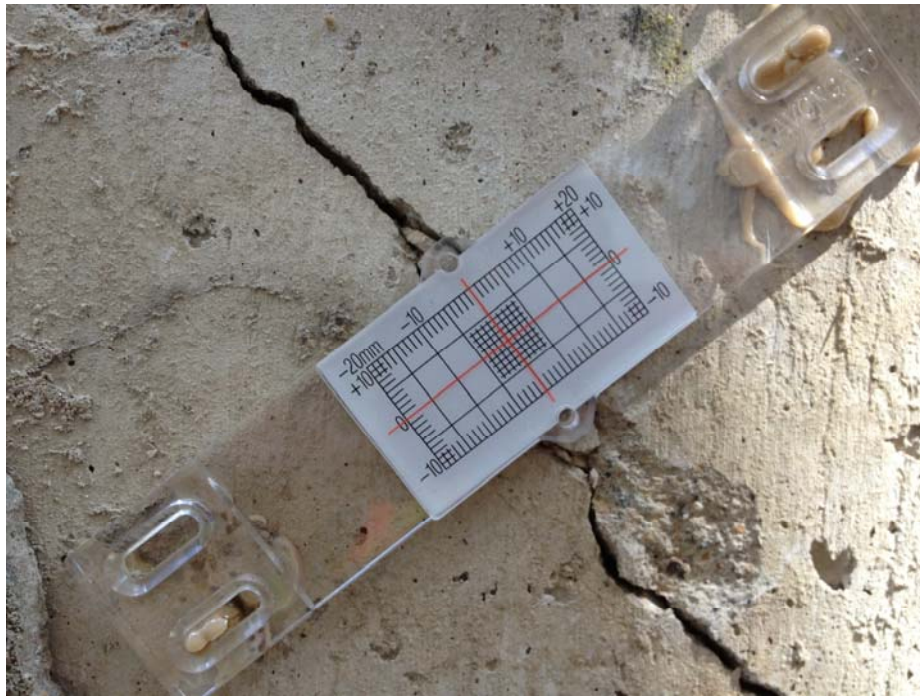
Photo F.5: Crack Meter Located on the West Face of the Retaining Wall Between 230 & 306 Sask. Cres. E. (CM3) (Aug 12, 2013)
