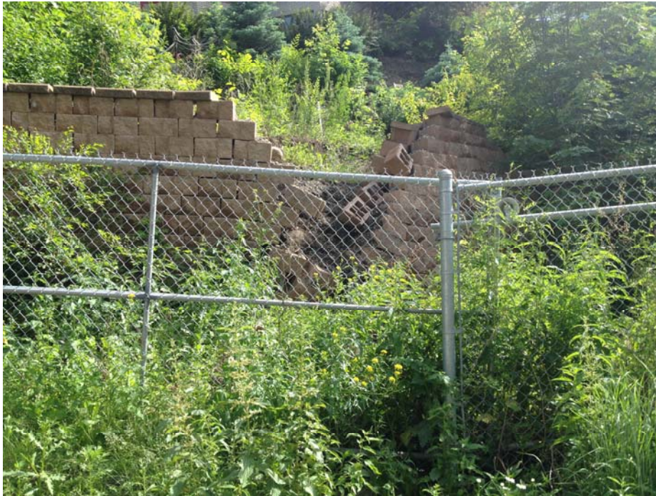
Photo C.19. Retaining Wall in Backyard of 237-239 11th St. E. (June 24, 2013)
