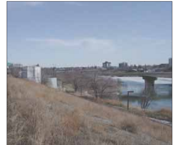
Undeveloped riverfront land and sewage pump station.
