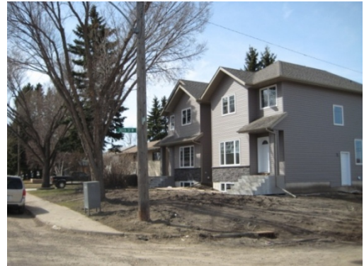
New semi-detached infill housing in Westmount
