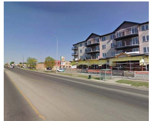
Arterial commercial with multi-unit residential in Calgary, Alberta
