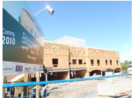
Bridgewater Hotel on 22 nd Street during construction
