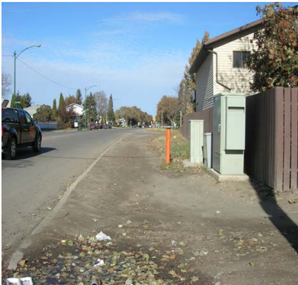
No sidewalk – Avenue P North to 23 rd Street West
