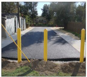
FIGURE 2.9 Infiltration Swale
