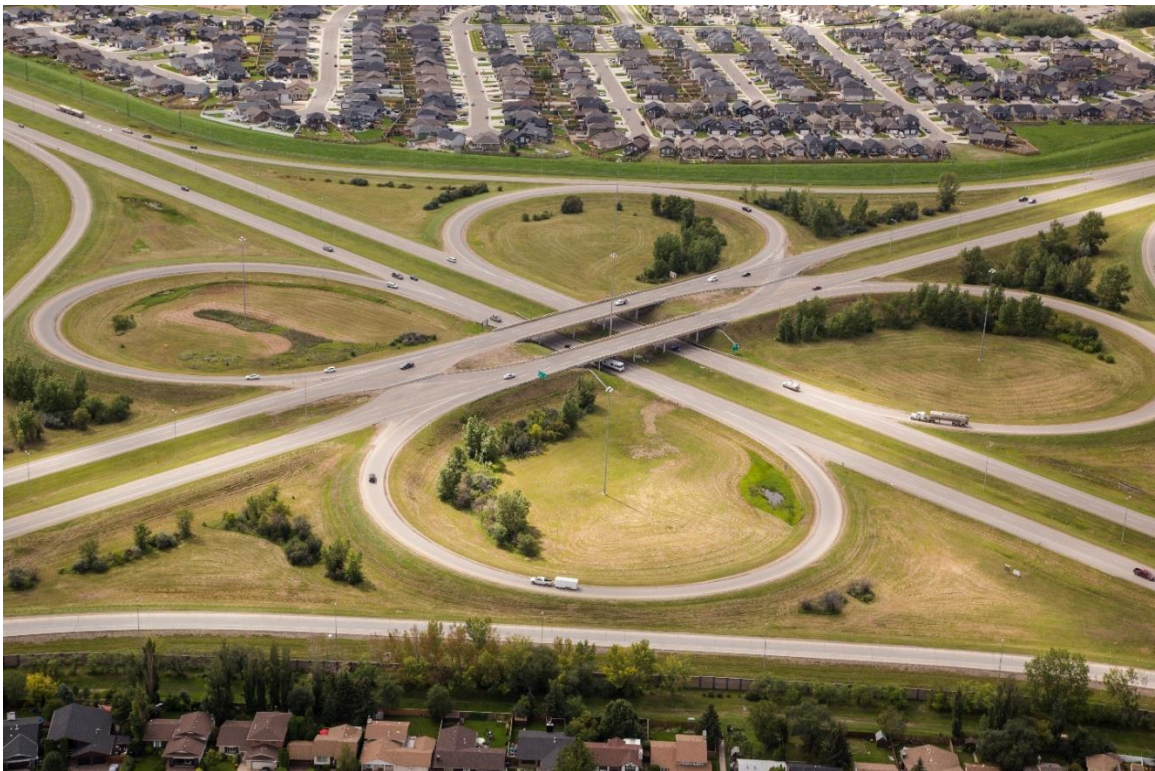
Figure 1.1: Existing Cloverleaf Interchange
