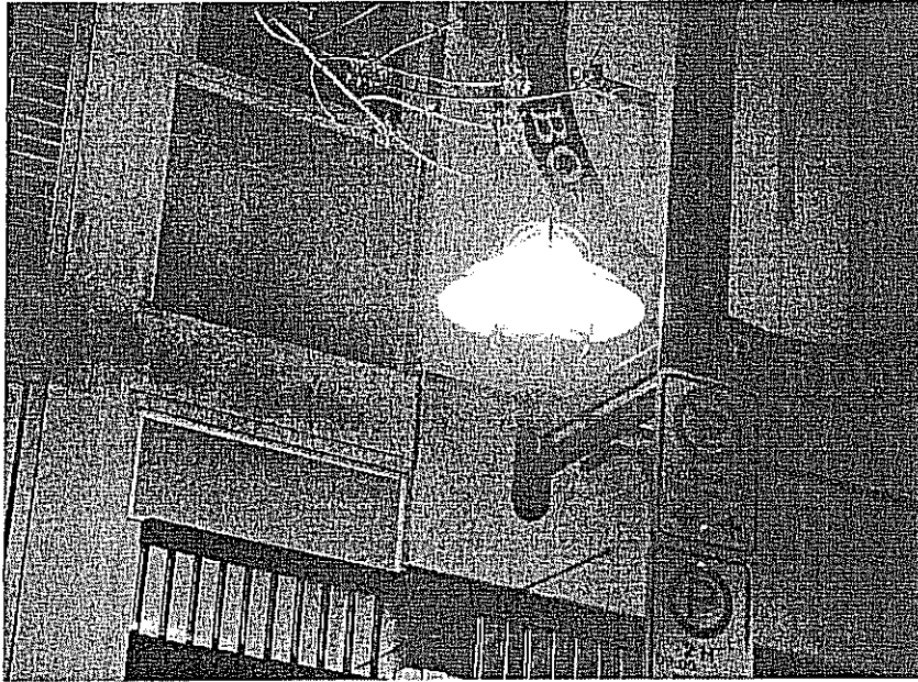
Figure 3: Semi-reflected lighting with open tops – globes in the Saskatoon Downtown Area. One-third of the light exits the top of these fixtures unimpeded, cause light pollution and light trespass into windows.
