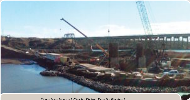
Construction at Circle Drive South Project
