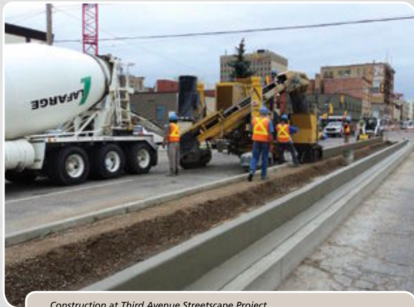
Construction at Third Avenue Streetscape Project
