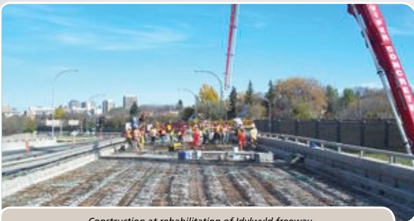
Construction at rehabilitation of Idylwyld freeway
