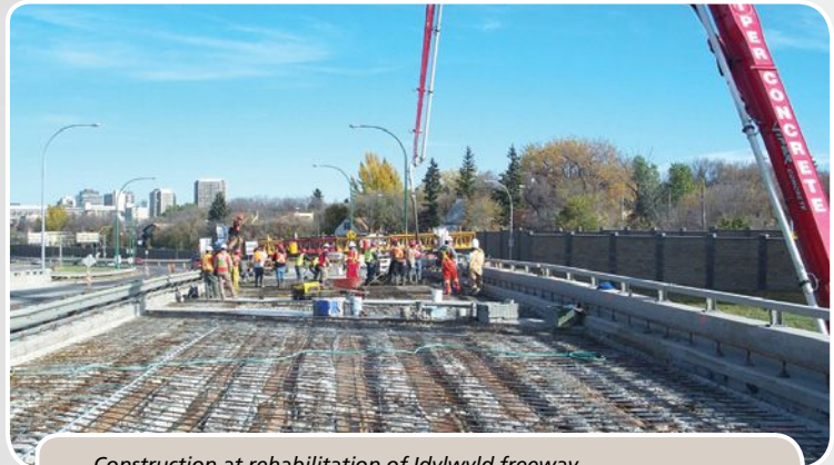
Construction at rehabilitation of Idylwyld freeway
