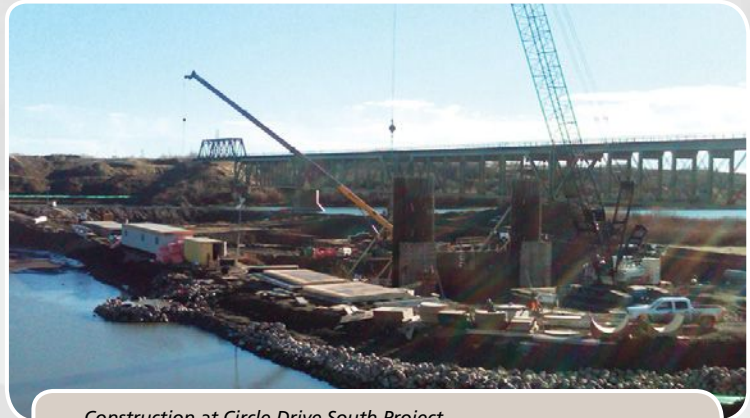
Construction at Circle Drive South Project
