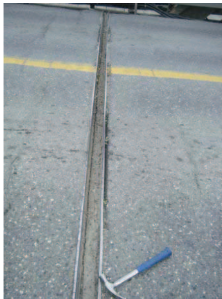
Photo 14 Joint at pier 4
