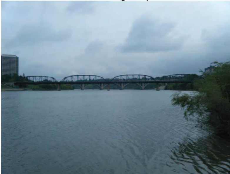
Photo 17 Elevation from upstream
