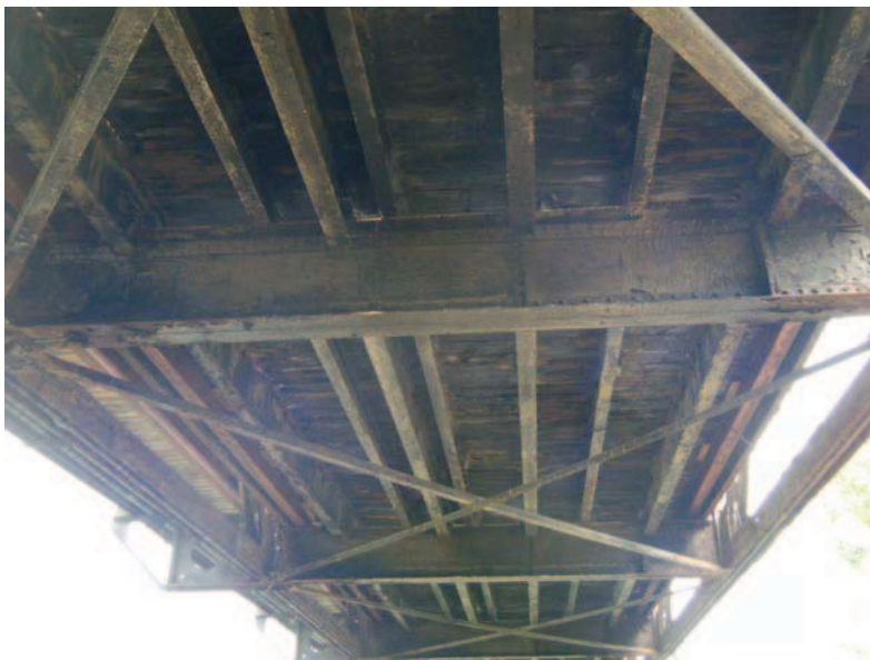
Photo 22 Typical shot of floor beam stringers and bottom chord bracing
