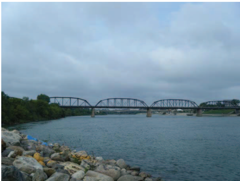
Photo 18 Elevation from downstream
