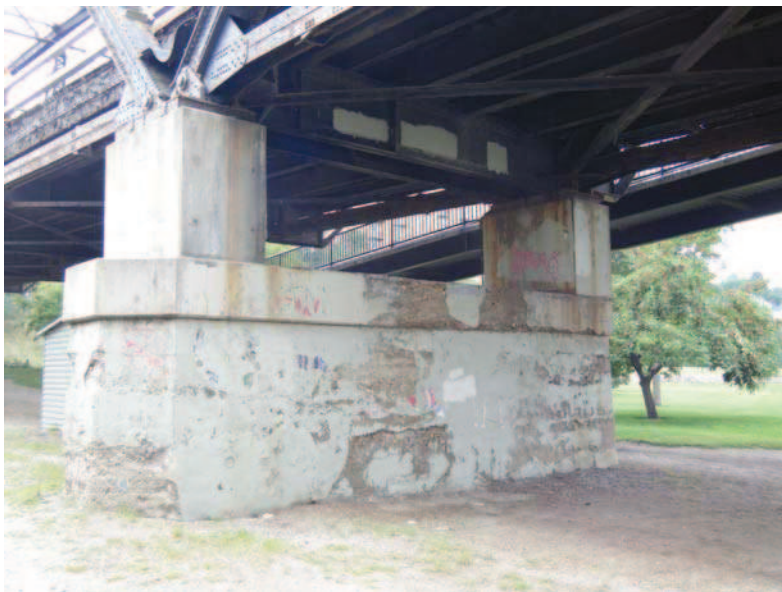
Photo 20 Typical shot of pier 1
