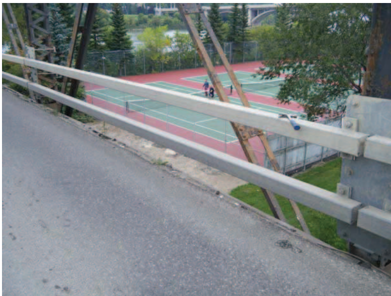
Photo 4 Typical railing RHS
