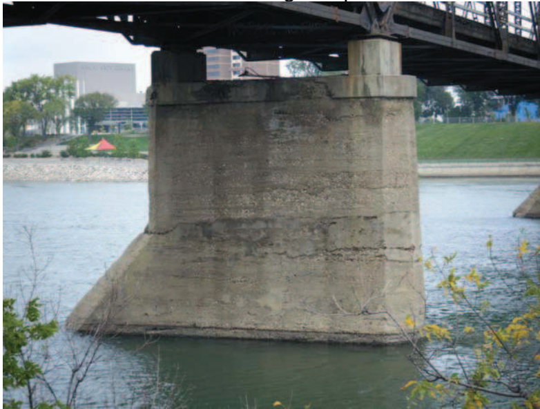
Photo 19 Typical shot of pier 2
