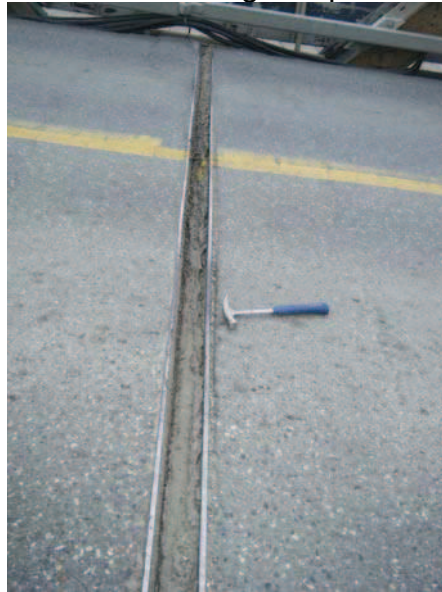
Photo 11 Deck joint at pier 2
