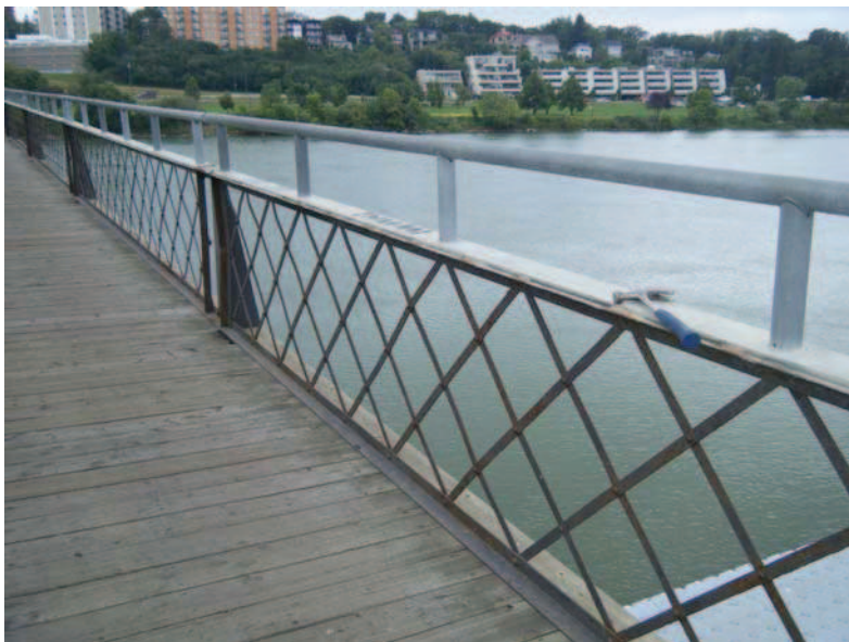
Photo 16 Typical shot of pedestrain rail
