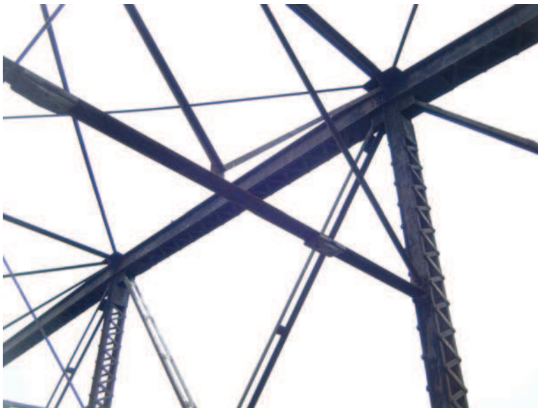
Photo 8 Typical shot of top chord
