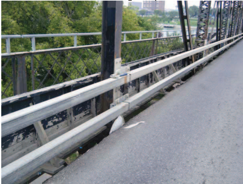
Photo 3 Typical railing, LHS
