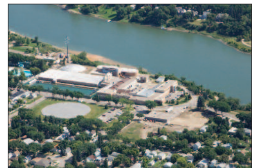
Aerial view of Water Treatment Plant, 2002
