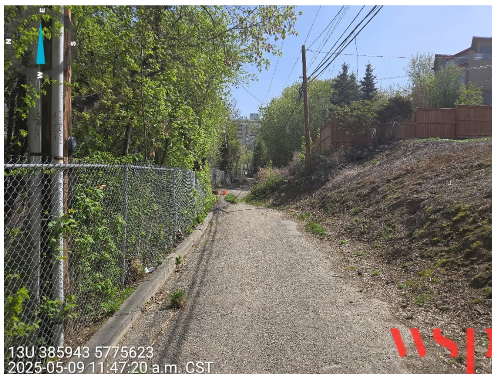
Photograph 2: Looking east down the back alley at the West Failure (May 9, 2025)
