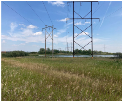
Figure 4-17: Powerline at the West Side of Chappell Marsh
