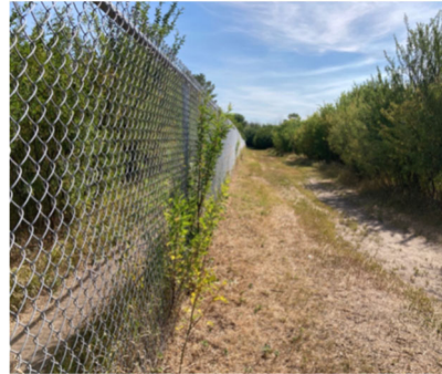
Figure 4-18: Fence at Northern Boundary of Off Leash Dog Area in Good Repair
