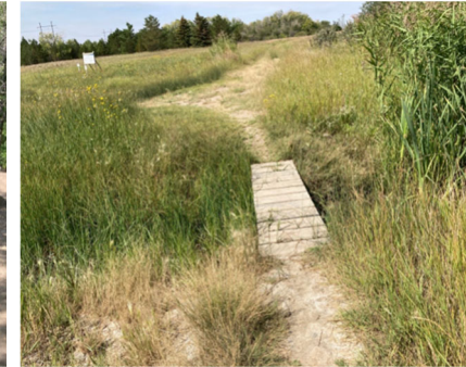
Figure 4-20: Small Bridge in RSBBA Path in Fair Condition
