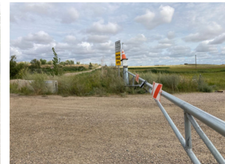
Figure 4-8: Snow Storage Facility Gate
