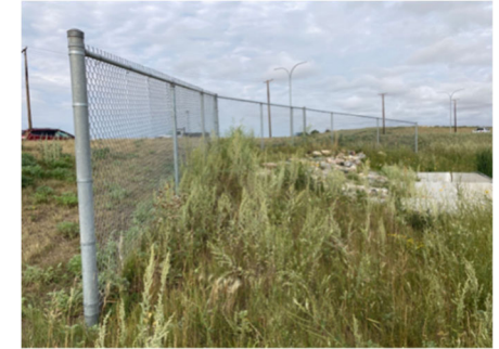
Figure 4-4: Chain Link Fence at Culvert
