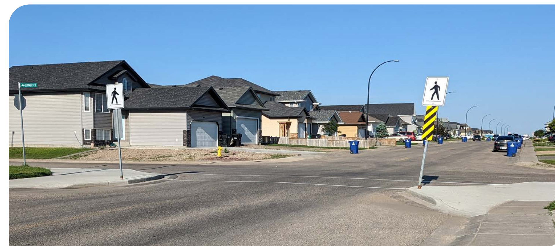
Curb Extension at McClocklin Road and McKague/Sumner Crescents
