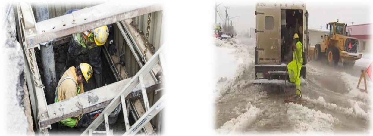
Figure 5.7 - Photos of Water Main Break Repair Work
