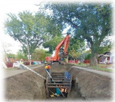
Figure 1.7 - Photo of Work in an Excavated Trench
