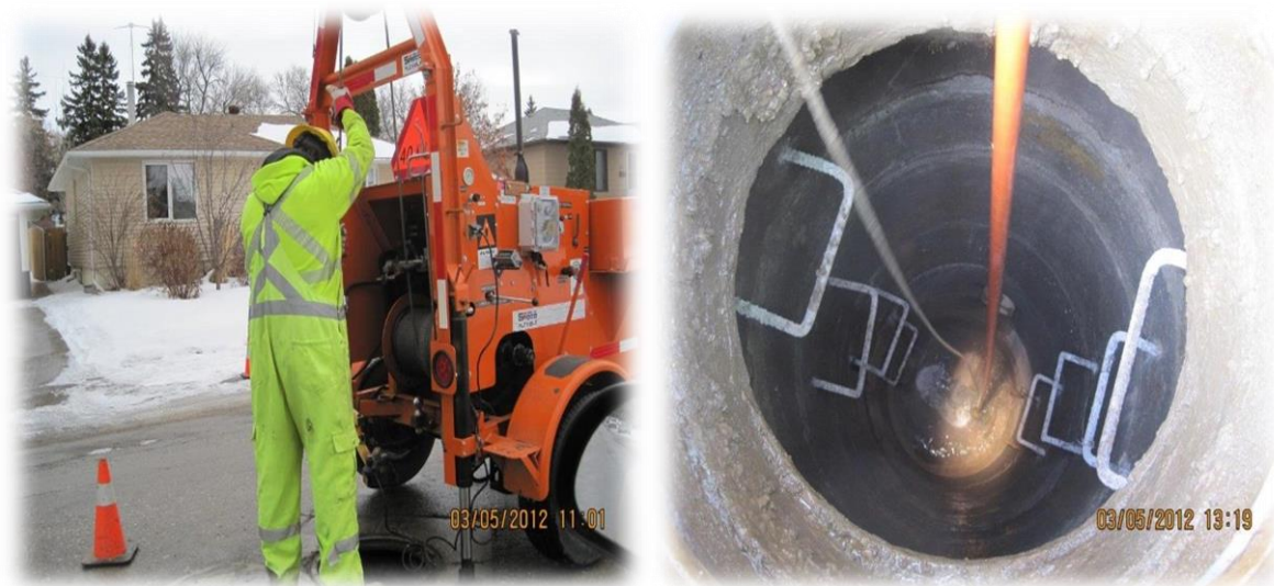
Figure 5.10 - Photos of Closed-Circuit Television Inspection Work
