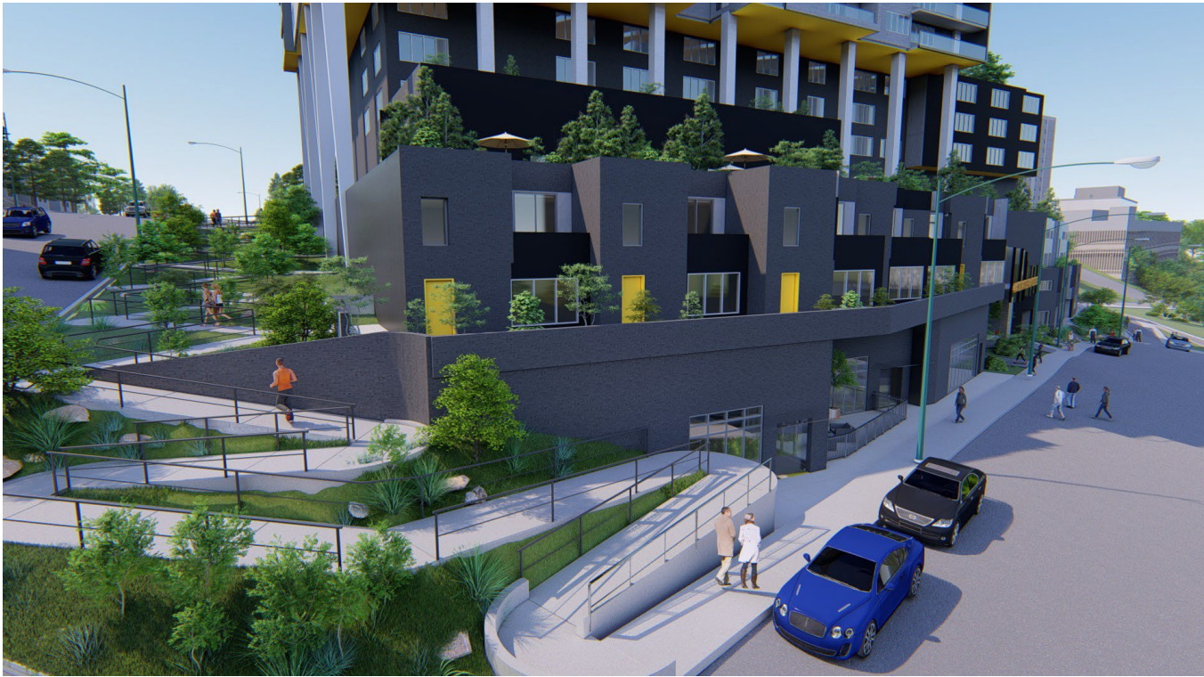
Barrier-free access (1:12 incline ramp) on Eastlake Ave.
