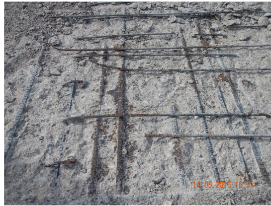
Severe corrosion on the reinforcing steel.
