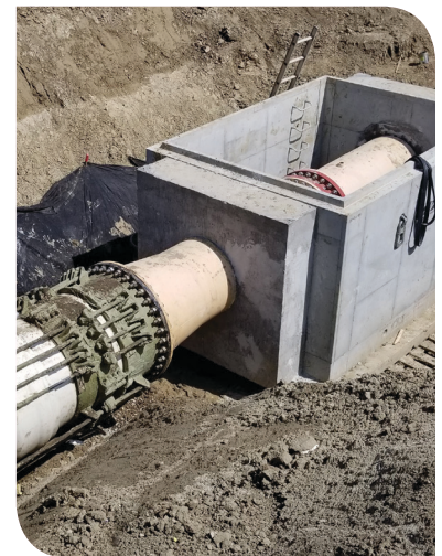
Primary water main and valve chamber
