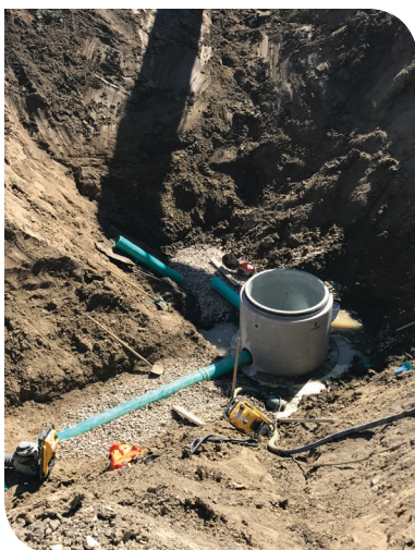
Sewer main and manhole construction
