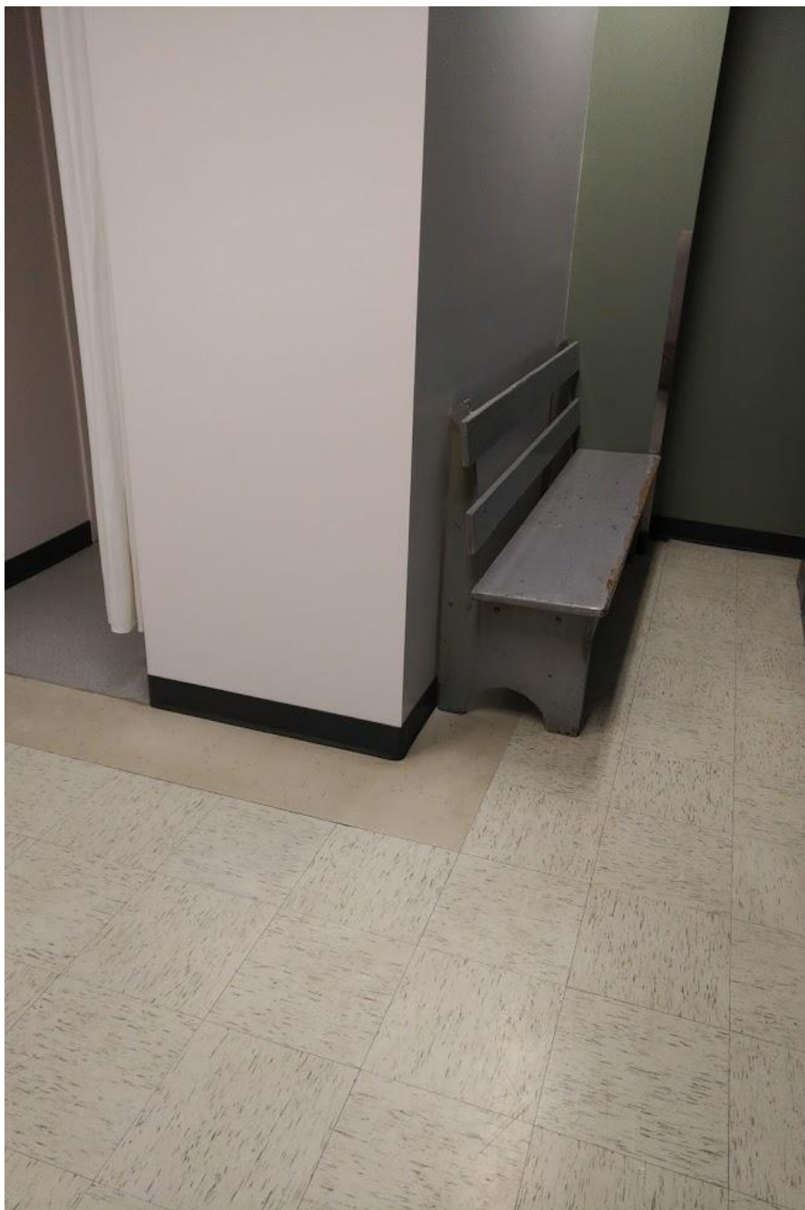
Photo 3: 210 Female Locker Room – 1' X 1' Floor Tile White w Grey Streaks. Asbestos Containing Material.
