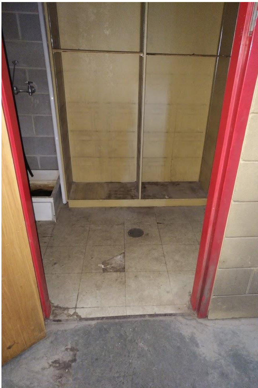
Photo 5: 122 Janitor Room – 1' X 1' Floor Tile Beige w Faint Grey Streaks. Asbestos Containing Material.
