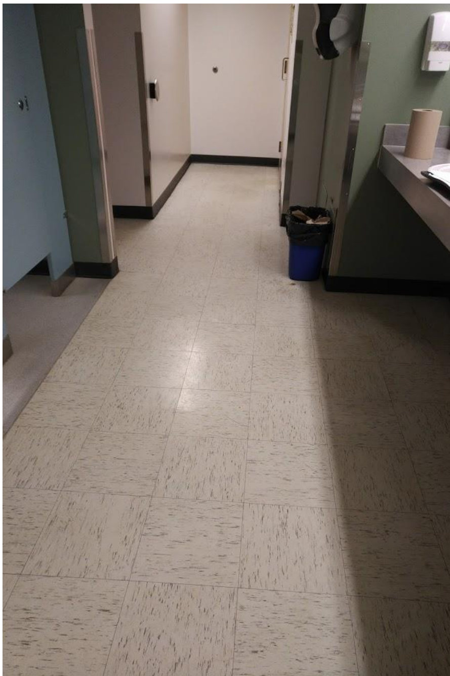
Photo 4: 209 Female Washroom – 1' X 1' Floor Tile White w Grey Streaks. Asbestos Containing Material.
