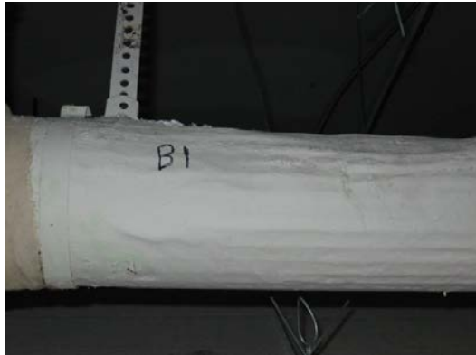
#1) Aircell Pipeline Insulation
